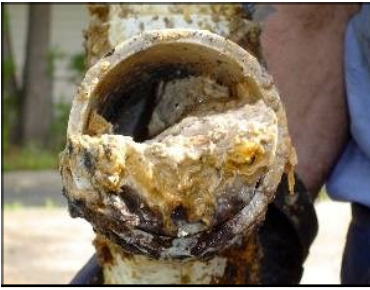
Picture provided by the Portland Bureau of Environmental Services, Portland, Oregon
