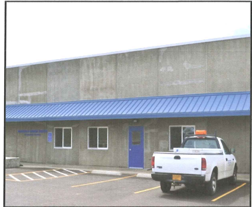
TREATMENT PLANT AT GRANGE RD. ROSEBURG, OR
